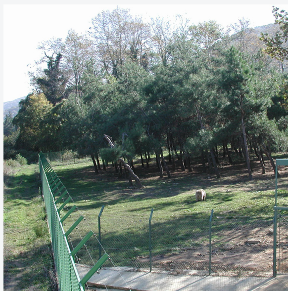
Figure 3. Net wire with electric fencing around perimeter.
