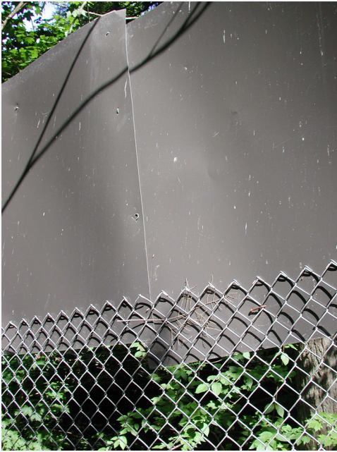
Figure 4. Heavy gauge metal sheeting mounted above chainlink.
